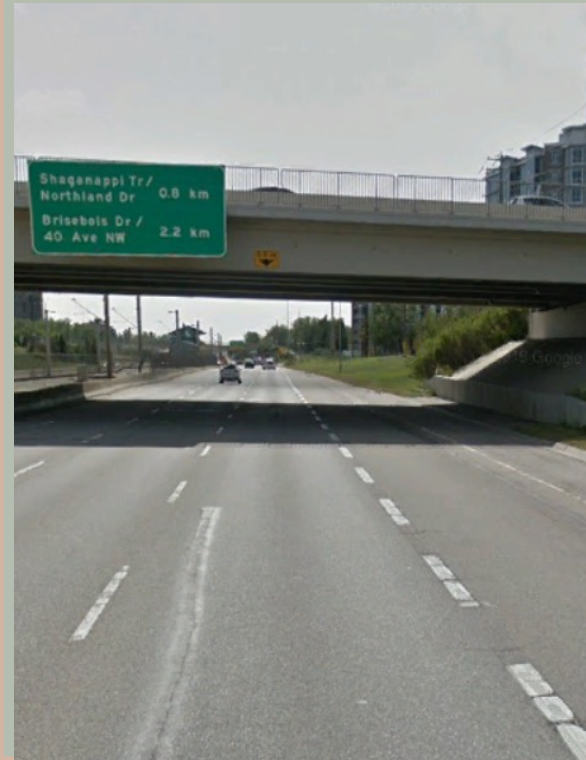
Highway with Overpasses
